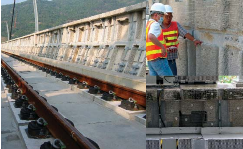
KCRC East Rail Extensions-Tai Wai to Shek Mun & Shek Mun to Lee On(TCC200 & TCC300) 東鐵支線大圍至石門，石門至利安
