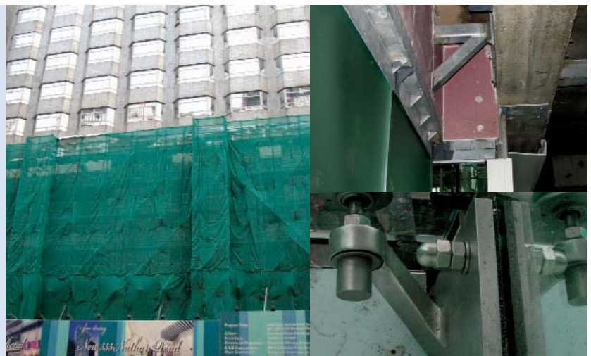
Kowloon Building, 555 Nathan Road A & A 九龍大廈
